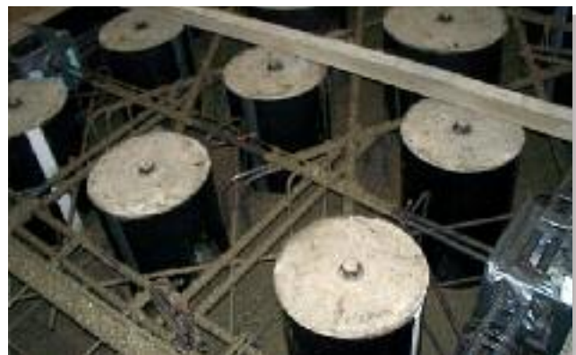
Steel alignment plates keep the cylindrical voids in place.
