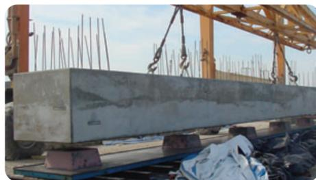
The typical pier cap is 55' long and weighs 8½ tons.
