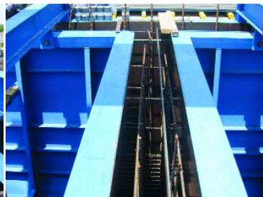
1. U-beam void with combination top tie/void hold down
