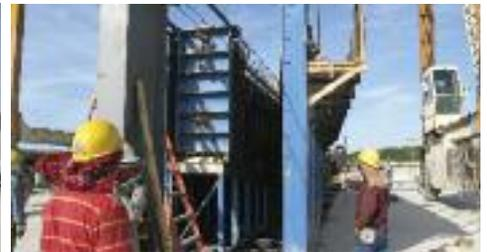
The picking points for the VLA are placed directly above the center of gravity so that sideforms hang vertically, optimizing handling of large, cumbersome sideforms. Some customers opt for a few sets of VLAs and use them on multiple sideforms. Others connect a VLA to each section of sideform and leave them in place, eliminating the need to store the VLAs and eliminating the attachment step from their set-up and stripping process.
